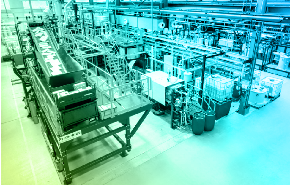
Shredder and beneficiation processing EV cells
